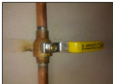
Shut Off Valve
